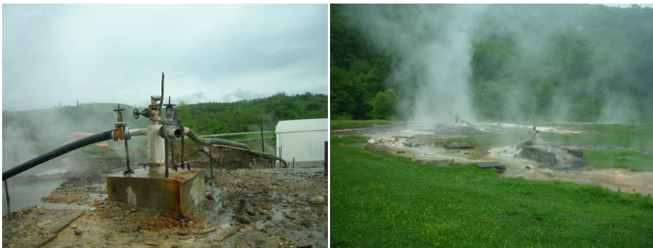
Fig. 5. “Tsaishi” and “Nokalakevi” thermal boreholes
