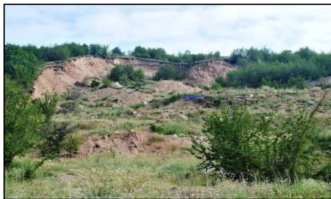
Fig. 3. A young active landslide formed on the body of an ancient landslide (photo by V. Boynagryan). It periodically blocks the highway and enters the flood-plain of the Aghstev river.
